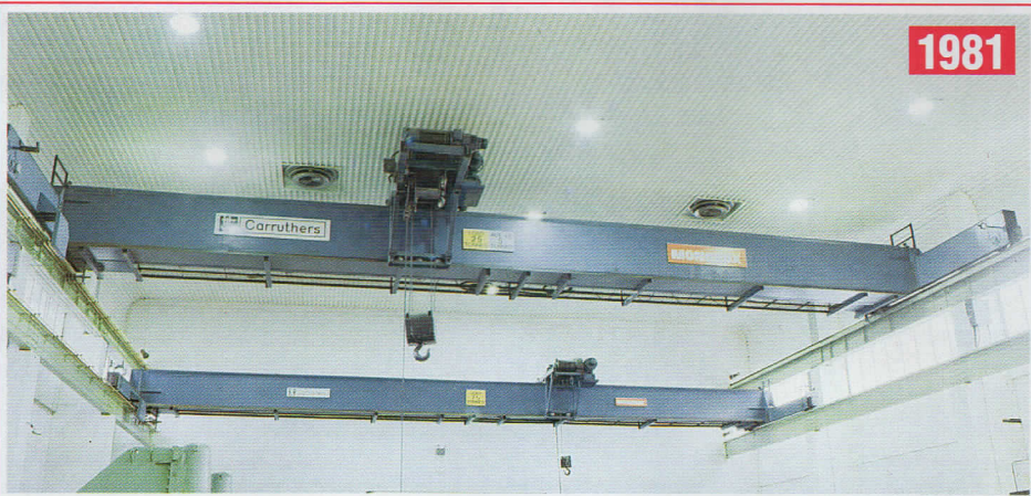
CARRUTHERS MONOBOX 25 tonne & 7½ tonne ELECTRIC OVERHEAD CRANES
